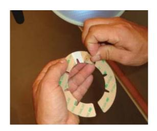
Place the foil under the arc so that it is centred and the middle cut-out clears the lamp's cooling vents.
