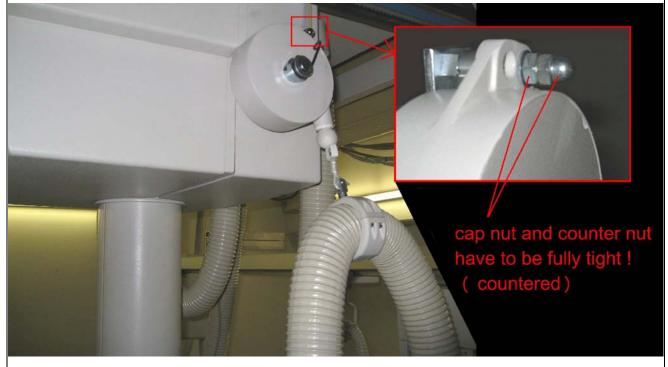
It is important, that both nuts (cap nut AND counter nut) are present and that they are fully tightened.
